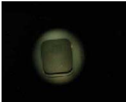
Clean exhaustgas channel
